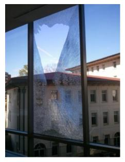
With an increase in spontaneous glass breakage incidents, the glazing industry is looking at new ways to make assemblies safer.
