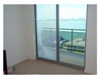
Safety glazings are commonly required for sliding glass doors, shower doors, and patio furniture. 'Safety glazing' generally refers to any type of glass that is engineered to reduce the potential for serious injury.
